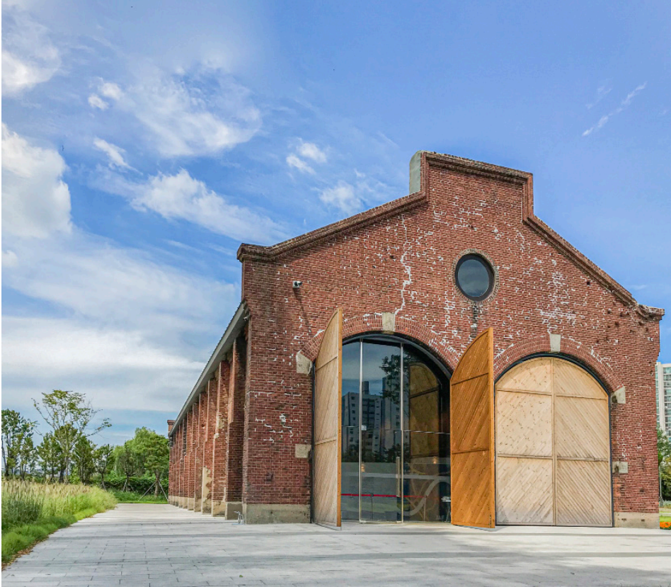
Vehicle Maintenance Depot at Jinju Station
